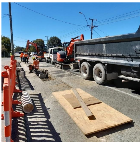
Image 4 - New water main High Street South
