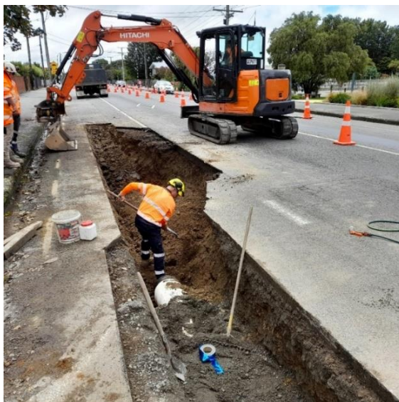
Image 3 - High Street South Water Renewal
