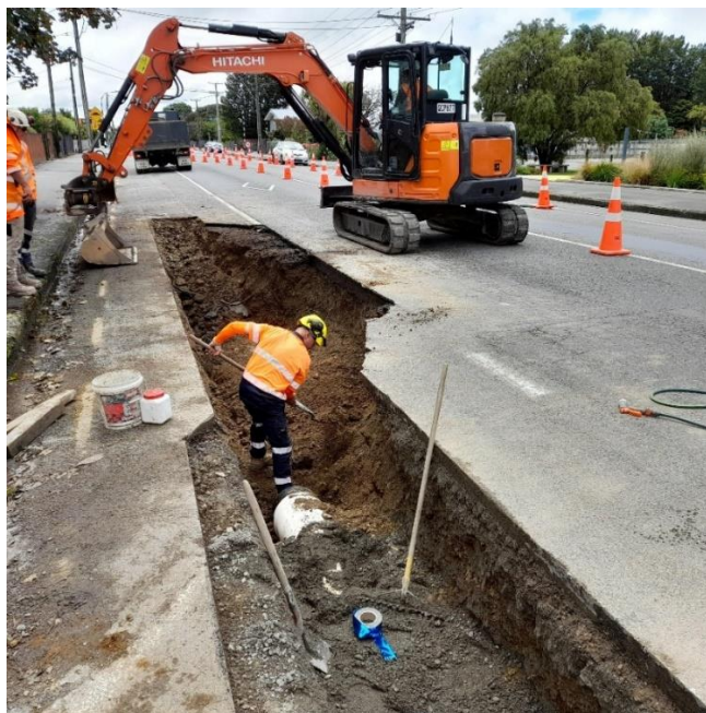
Image 3 - High Street South Water Renewal (1)
