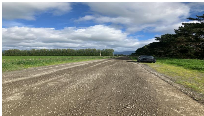
Unsealed road grading and metalling
