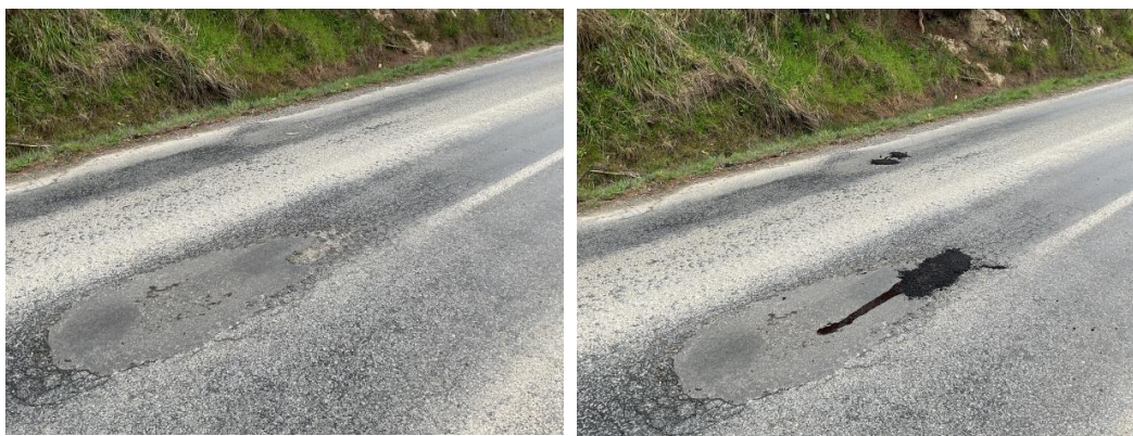
Pothole repairs
