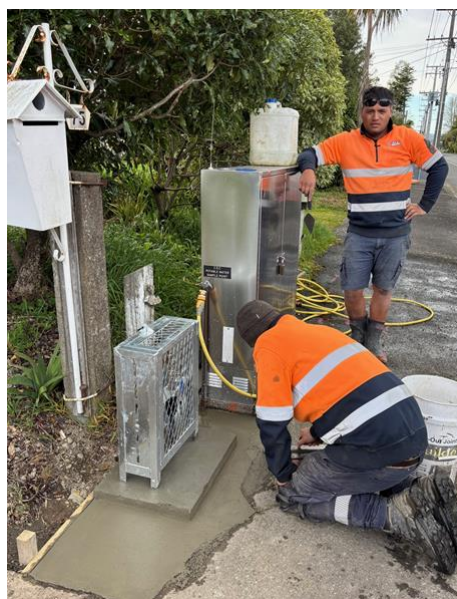
Image 4: RPZ Backflow Preventers being installed
