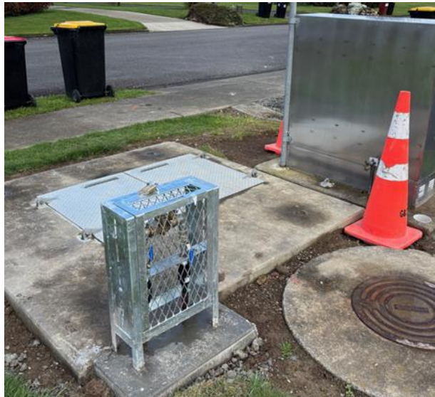
Image 5: New RPZ installed
