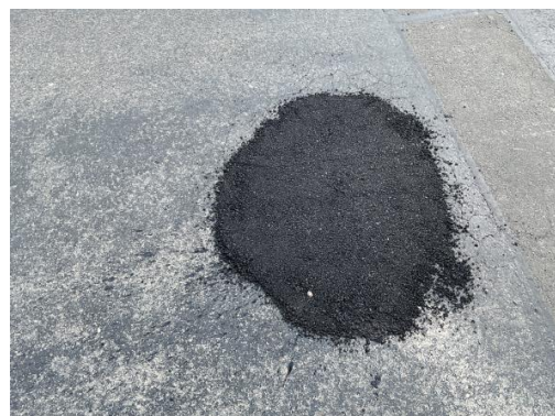
Pothole repaired
