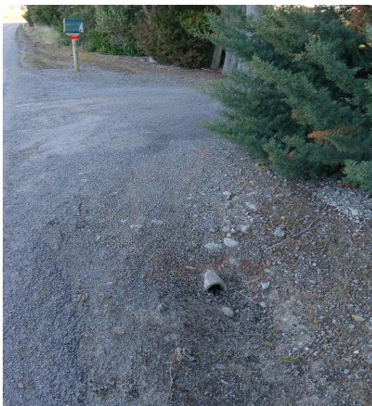
Figure 5 Photos of roadside drains, eastern side, left- undersized culvert, right-drain beside drive
