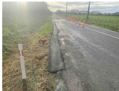
Edge break repairs on Carters Line Road
