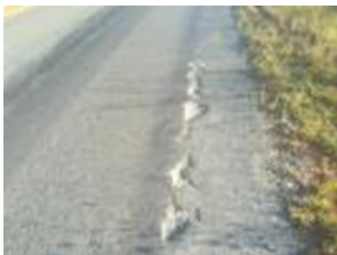
Pothole repaired on White Rock Road
