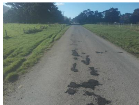
Pothole repaired on Hururua Road
