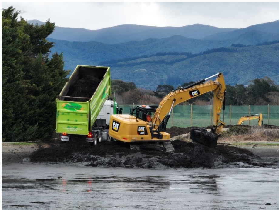
Image 14 - Sludge Removal
