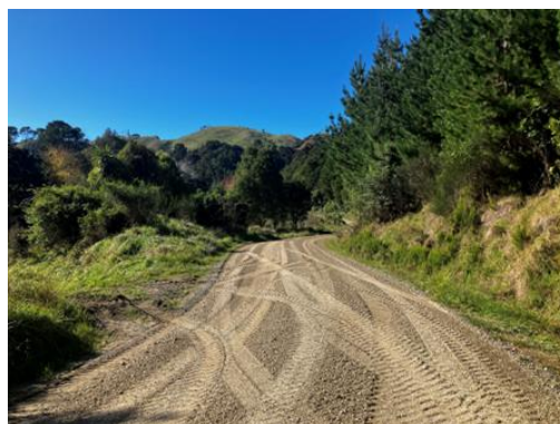
Unsealed road grading and metalling on Kaiwhata Road
