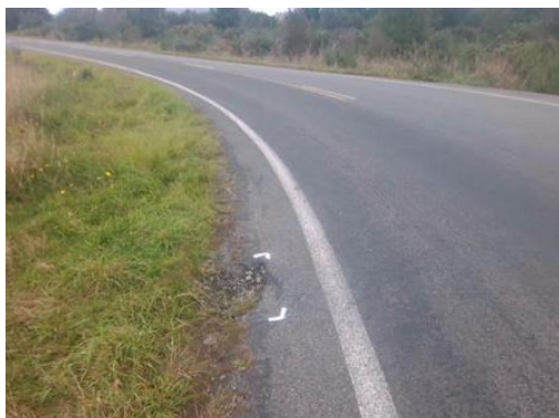
Edge break repairs on Greytown Woodside Road
