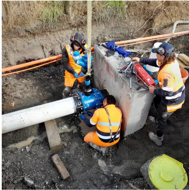
Image 7 - Brooklyn Water Main Replacement – Linking to old main
