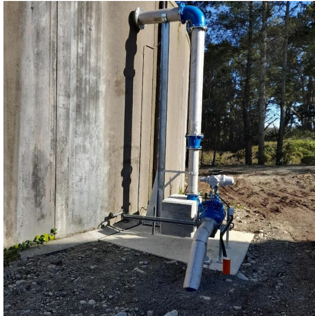
Image 5 - Inlet pipe to reservoir
