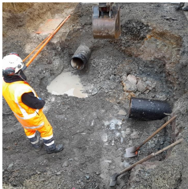
Image 6 - Brooklyn Road Water Main Replacement Linking to old main
