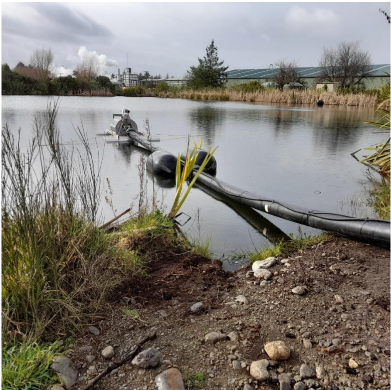
Image 3 - Pump Inlet System (3)
