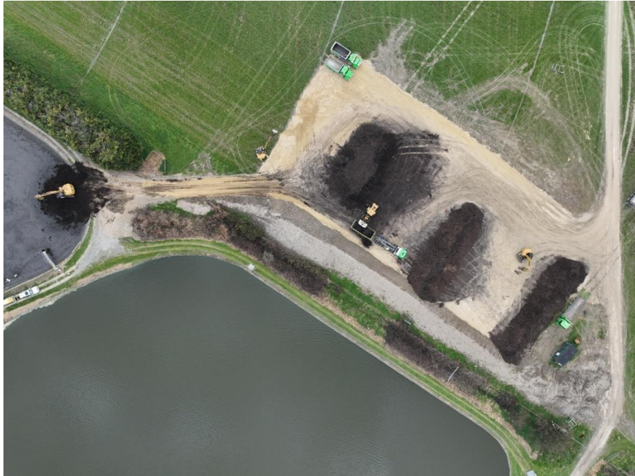
Image 13 - Sludge Removal (2)
