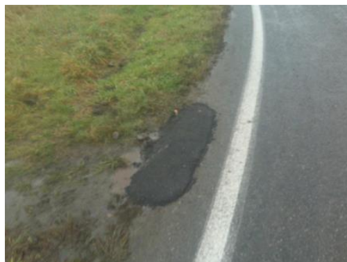
Edge break repairs on Greytown Woodside Road
