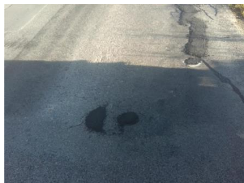
Pothole repaired on White Rock Road
