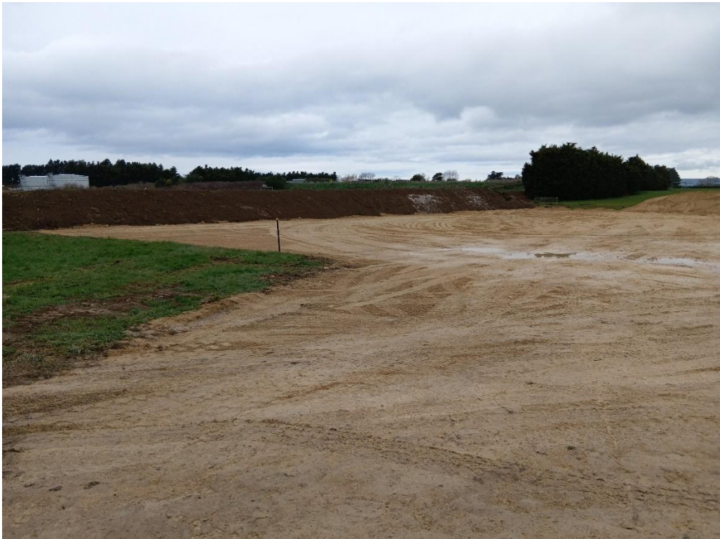
Image: bunded lime pad 50% complete
