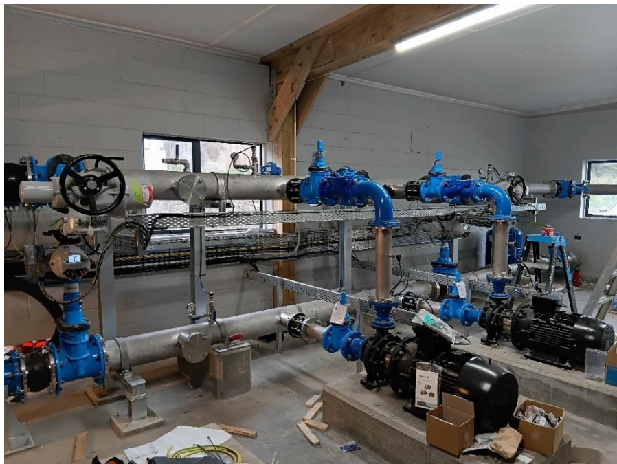
Image: New pump stations in the final stages of assembly
