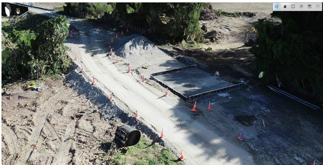
Image 8 - Ford under construction
