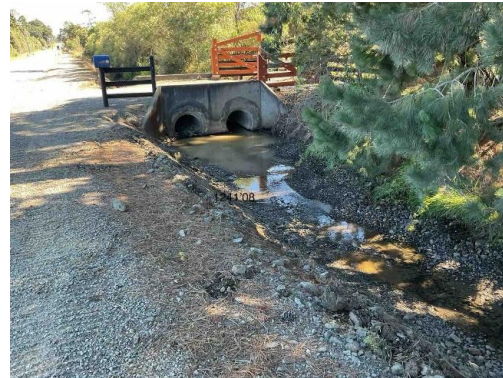
SWC (Unlined) - Clean, Swale Drain around culvert at Underhill Road (Extension@Wakefield)
