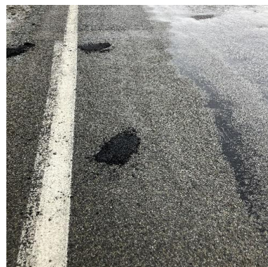
Pothole repaired on Cape Palliser Road
