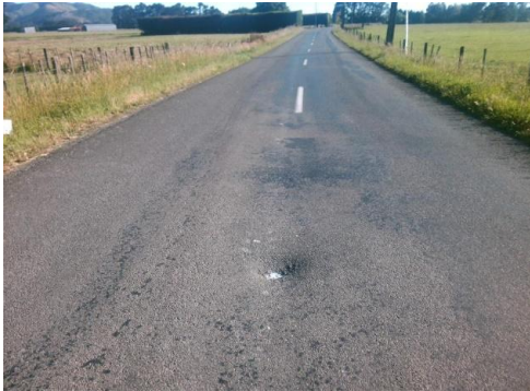
Pothole repaired on Watsons Line
