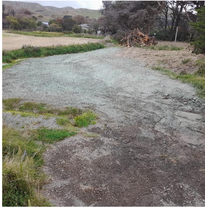
Image 6 - Stage 4 Complete with Hydroseed
