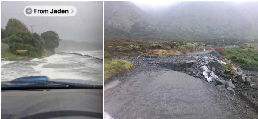
Waves breaking on the road at Te Kopi. Carriageway wash out at RP 36926 ford crossing before light house.
