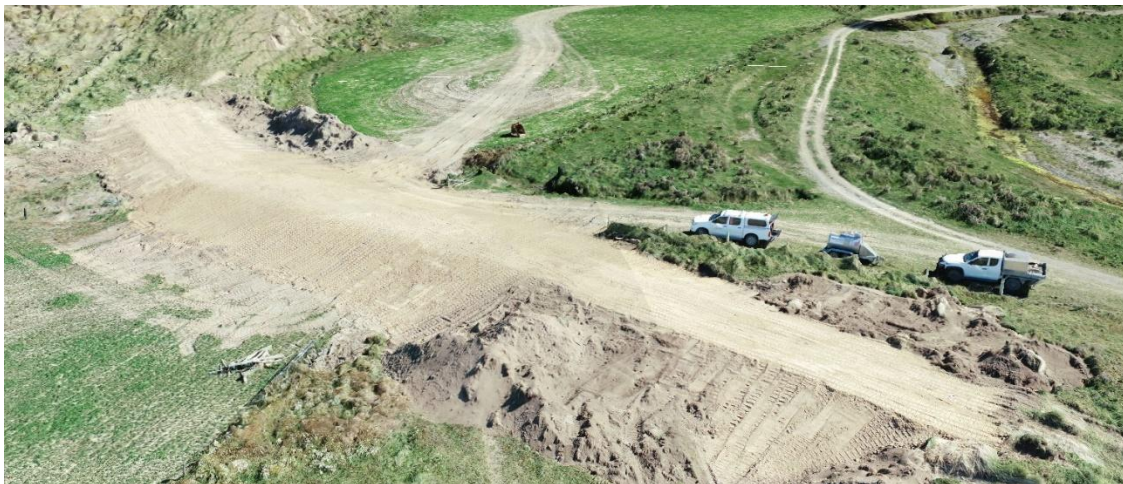
Image 7 - Bund before topsoiling
