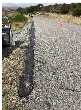
Edge break repairs on Gladstone Road
