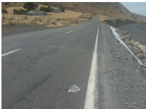
Pothole repaired on Cape Palliser Road
