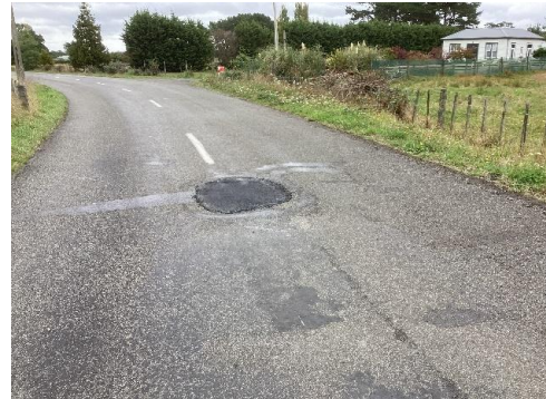
Pothole repaired on Watsons Line
