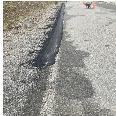
Edge break repairs on Cape Palliser Road
