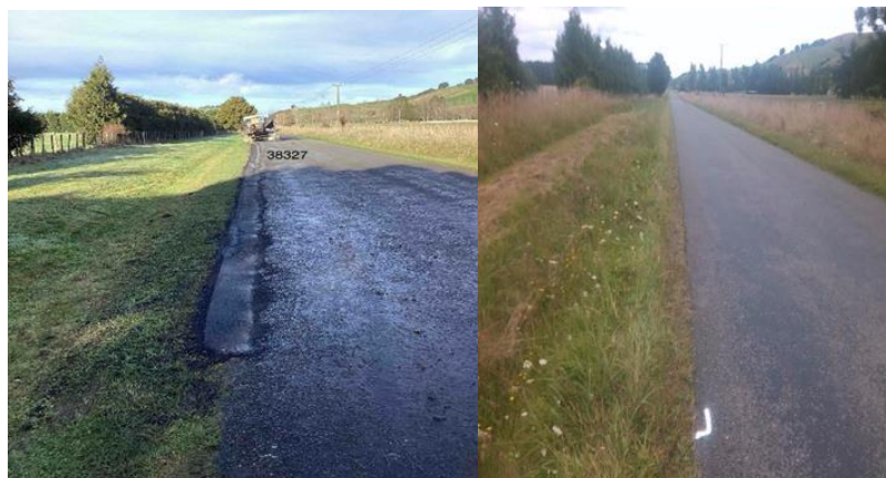
Edge break repairs undertaken on Haringa Rd
