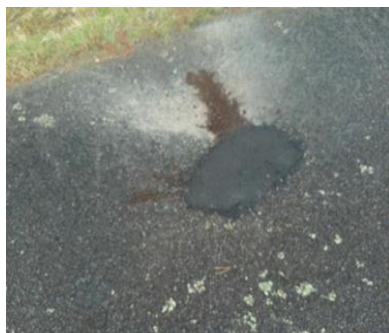
Potholes repaired on Hururua Road
