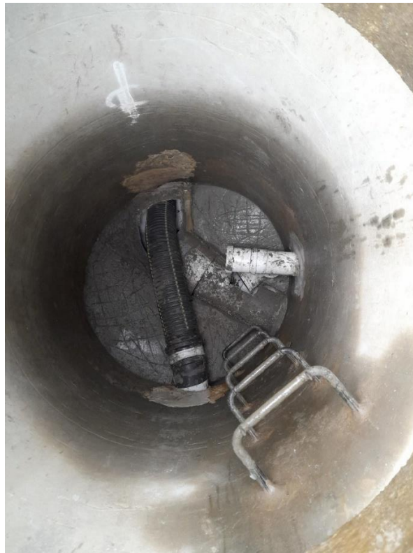
Figure 1- Typical cut over process to keep the sewer live
