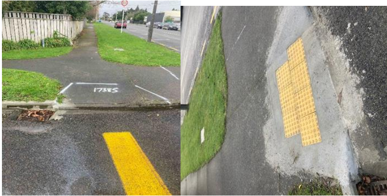
Tactiles installed on Wakefield St
