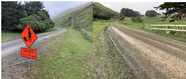
Unsealed road grading on Glenburn Rd
