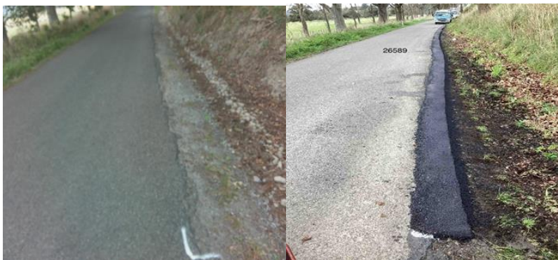
Edge break repairs were undertaken on Te Kopi Rd
