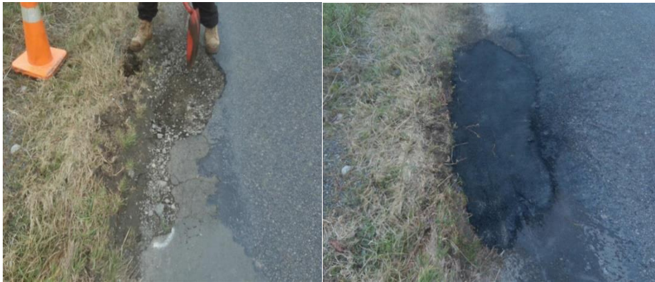
Image – edge break repair
