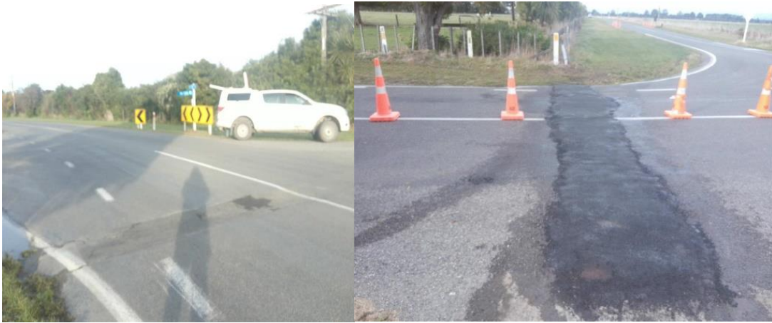
Image - Trench levelling
