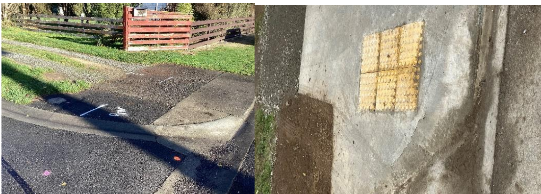
Image – installation of new tactiles on Brooklyn Road
