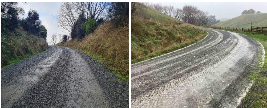
Image - Unsealed road grading on Ruakiwi Rd
