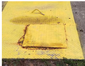
➤ Metal plate needs securing
