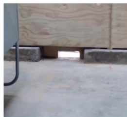
➤ Concrete flooring and drain holes to the outside of the building make for ease of cleaning and disinfecting
