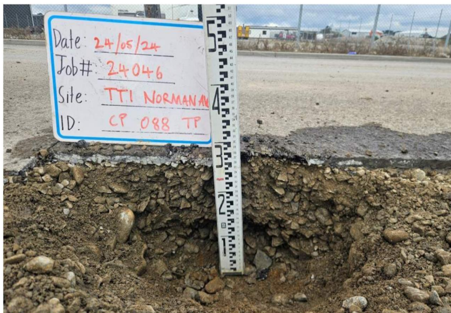
Figure 4 - Existing road foundation on Norman Avenue
