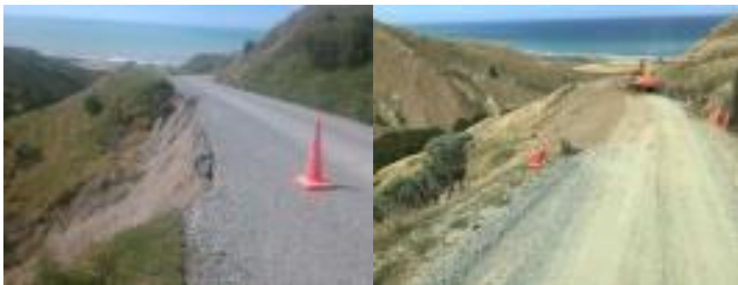
Dropout repairs on Glenburn Rd
