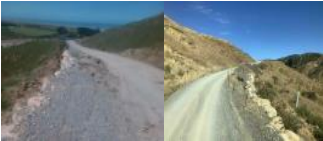
Dropout repairs on Te Wharau.
