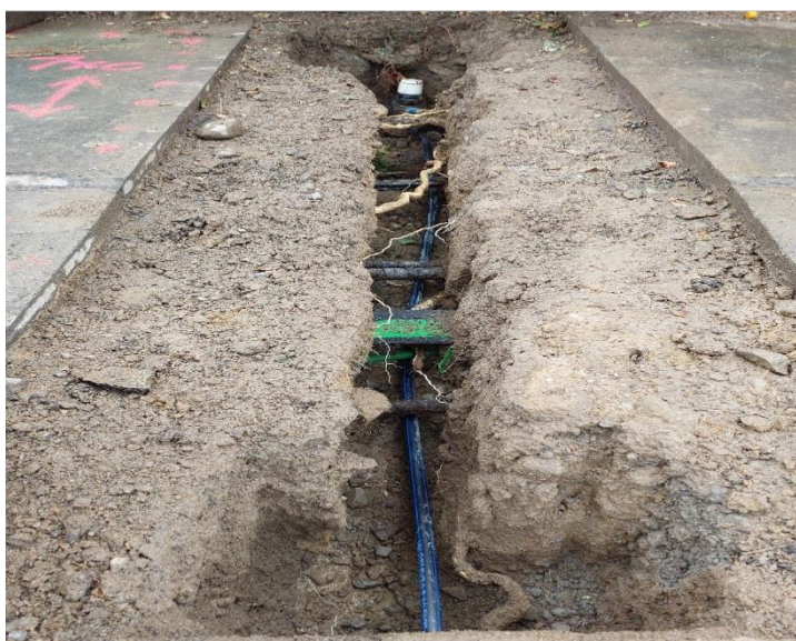
Underground services visible in footpath
