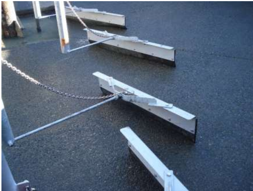
Scrapers in new condition after the last maintenance was completed on the clarifier.
