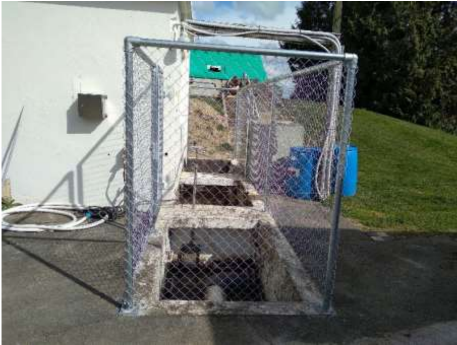
New Fencing and Gate around the Open Channel into the Pump Room.
