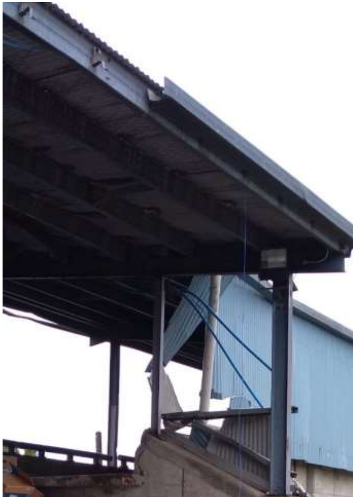
Showing damaged Cladding and missing Spouting.
