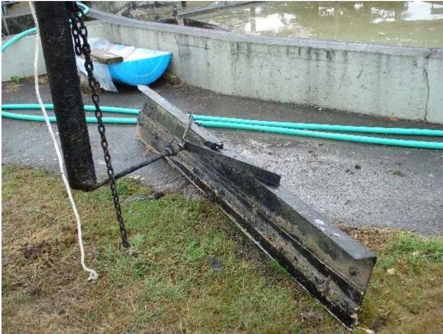
Likely condition of the scrappers with worn rubbers and corroded steel work.
