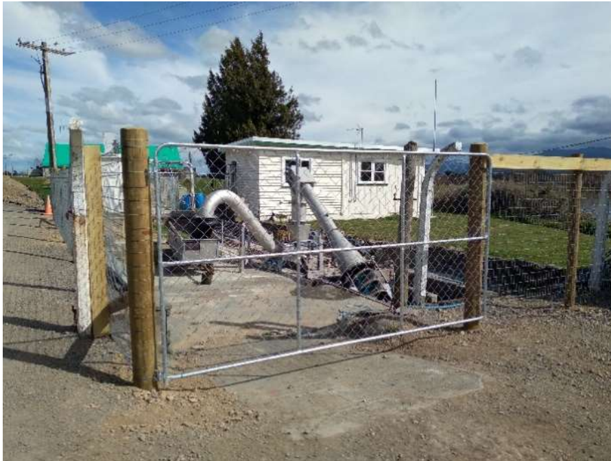
New Truck Entry Gate.
