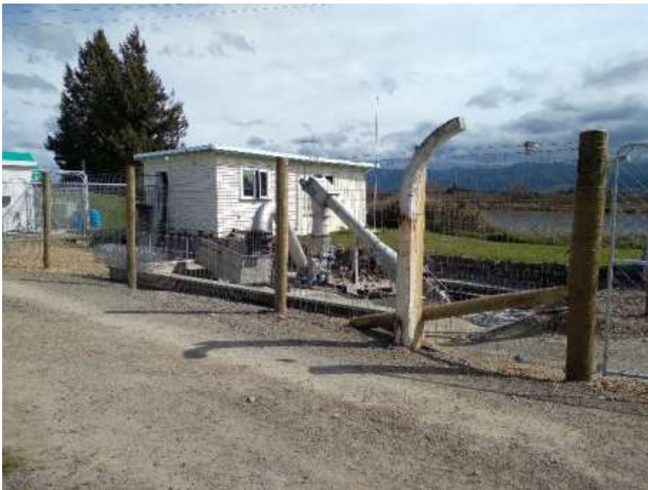
Fencing Around the Incoming Channel.
