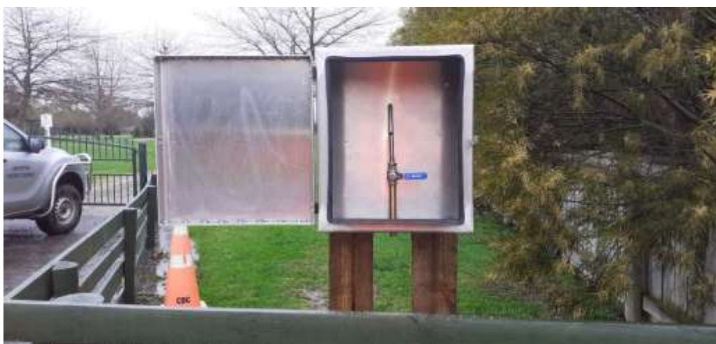
Plimsol St and Sparkes Park – Boxes mounted ready for Plumbing.
