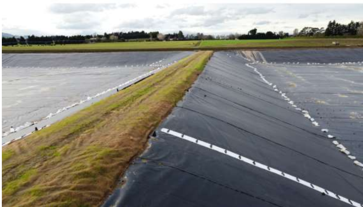
Figure 2: Topsoil and grassing of crests
