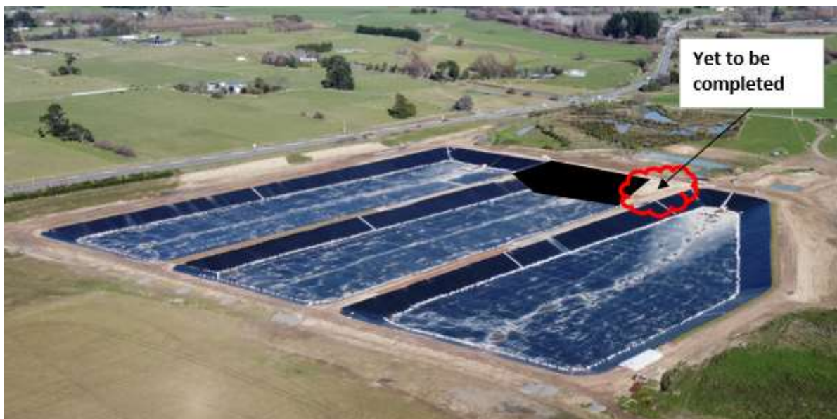
Figure 1: Southern Dam Wall near completion
