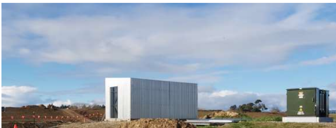
Figure 3: Control Building and 300KVA Transformer.
