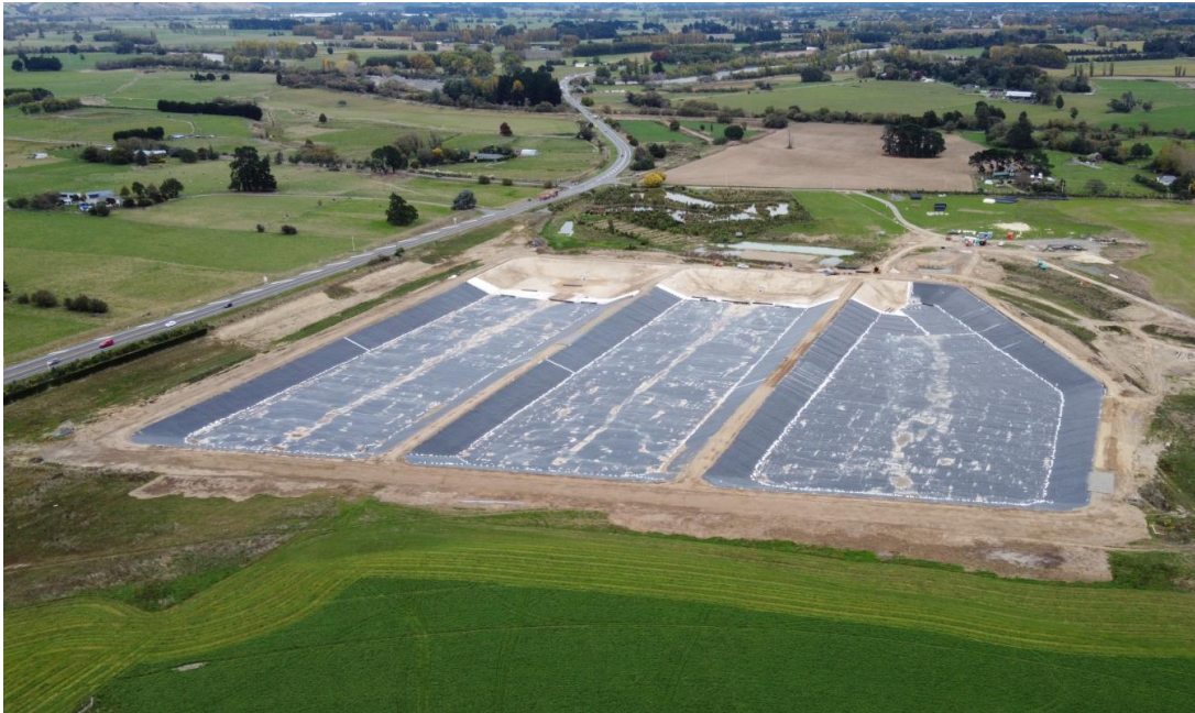
Figure 1 – 20 April 21 – All Pond's now have a majority of their liners installed
