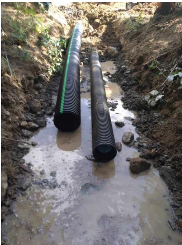
Figure 4: Pipe extension attached to both the culvert and replaced scour valve outlet.
