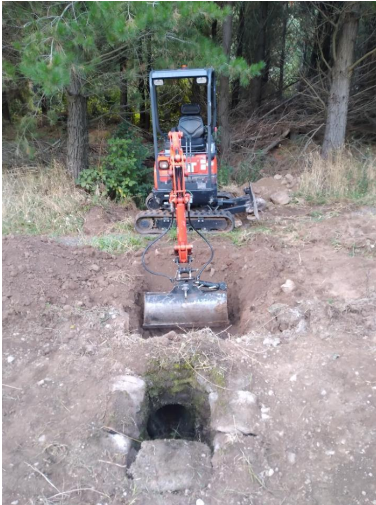
Figure 2: The foreground shows the culvert sump with the outlet of the culvert seen in the picture.
