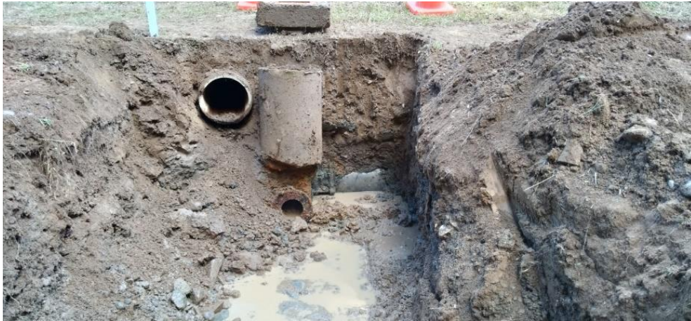
Figure 3: A view of the culvert (top left) and the scour valve visible at the base of the trench.
